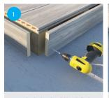
Two pilot holes should be drilled at every joist, leaving a gap of at least 50mm from both the beginning and the end of the trim.
